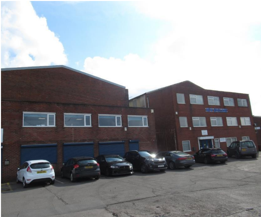
View of the Front Elevation
