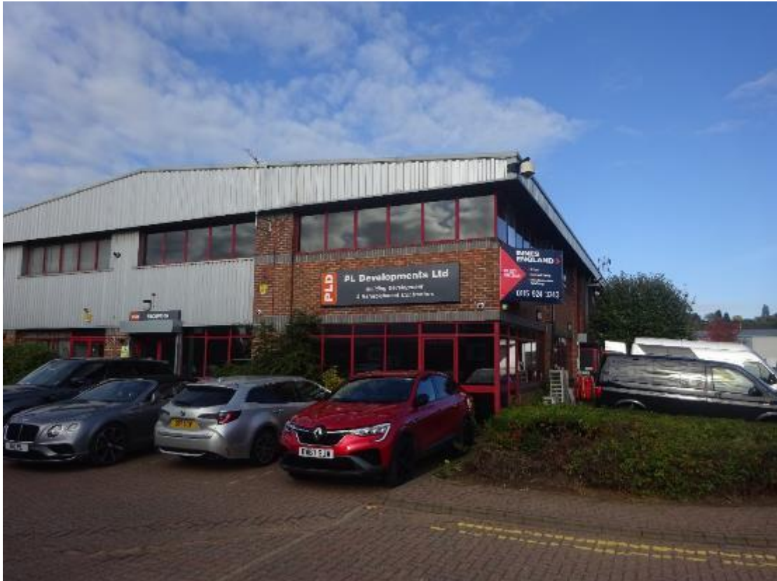
View of the Front Elevation
